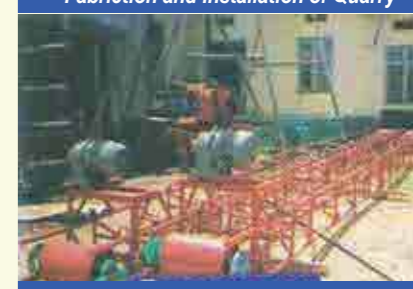
Fabrication of Conveyors,
