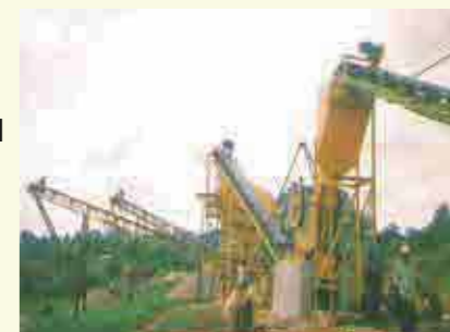
Fabricition and Installation of Quarry
