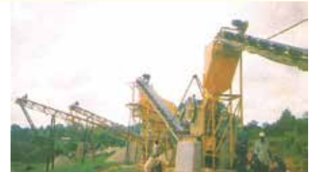
Installation of Quarry Plant
